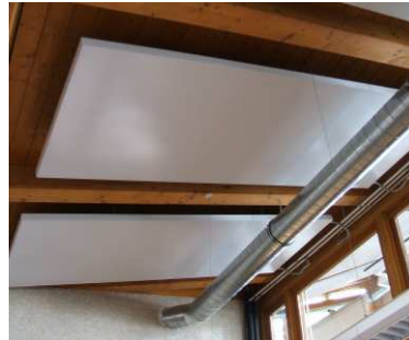
Figure 11: Chilled ceiling elements in a school in Butzbach, Germany (picture source: Fraunhofer ISE)
