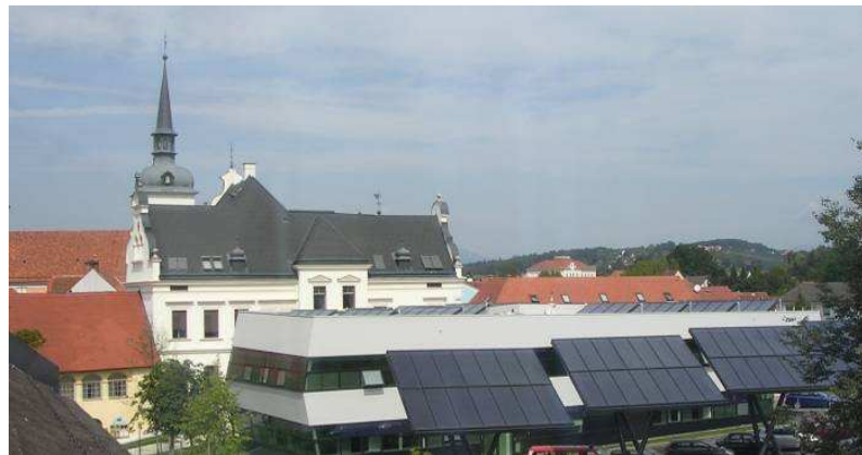
Figure 7: Double glazed flat plate collectors at the town hall / service center of the city of Gleisdorf, Austria (picture source: AEE INTEC)
