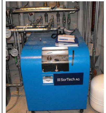
Figure 10: 7.5 kW adsorption chiller (picture source: SorTech)
