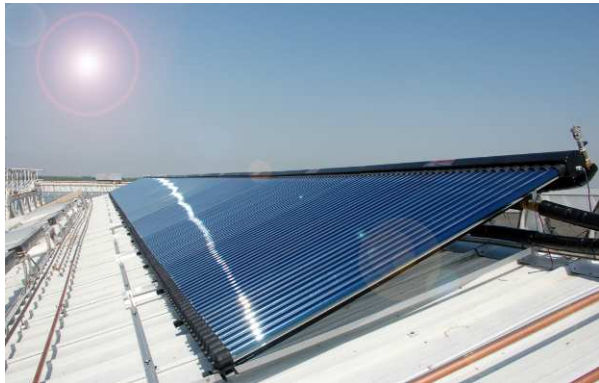
Figure 6: Evacuated tube collectors at Venice Marina (picture source: Climatewell)
