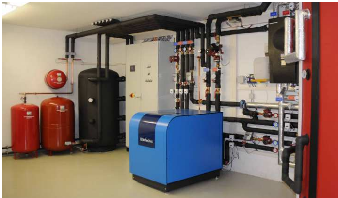
Figure 12 - Solar heating and cooling system in a municipal administration building in Vienna, Austria (picture source: SOLution)
