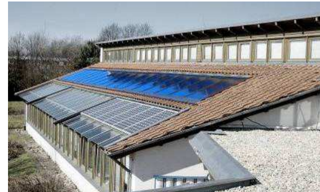
Figure 5: Flat plate collectors (picture source: Sonnenklima)
