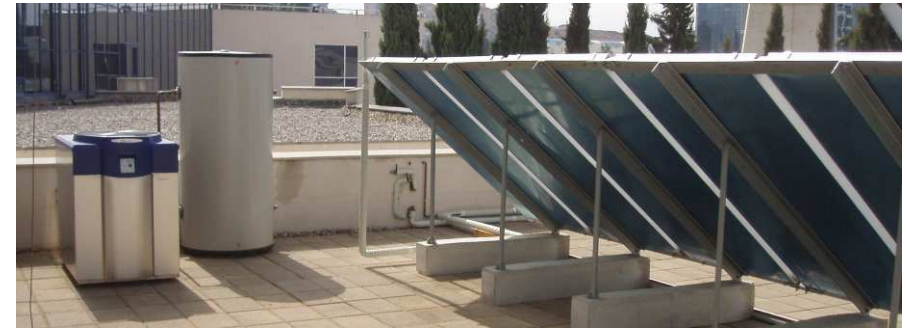
Figure 13 - Solar cooling system installed on a roof in Granada Spain (picture source: IKERLAN)
