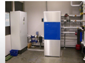
AKM Installation Mannheim, district heating
