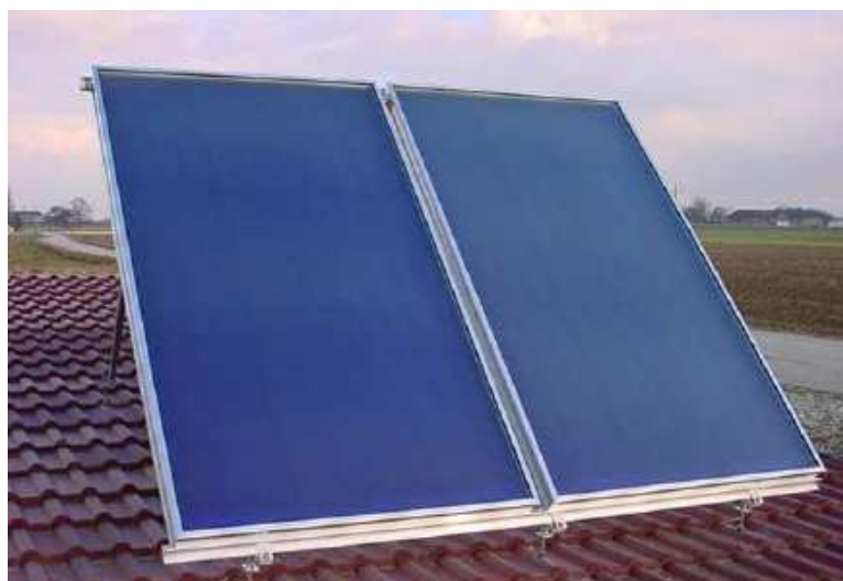
Figure 3: 2 Flat plate collectors, each with 2.7 m 2 surface area
