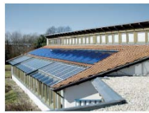
Illustration Solar installation for the solar cooling at the Centre for Environment and Technology (CET) in Osnabrück. Source: St. SonnenKlima, 2005.
