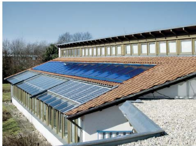
Illustration: Solar installation for the solar cooling of the Centre for Environment and Technology [CUT] in Osnabrück.
