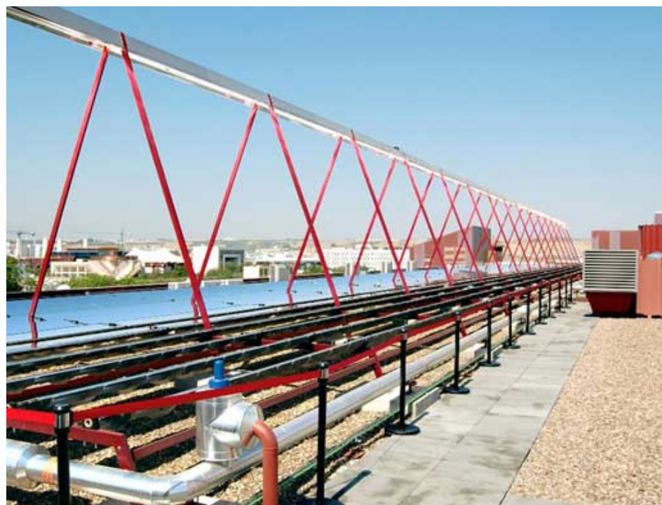
Photo: Climatization of a building of the University of Sevilla. Chiller: Double-stage BROAD BZH 15 IX, China. Source of power: 352 m 2 linear-concentrated Fresnel collectors (Mirrox, Germany). Reverse chilling: Cooling tower. Cooling: cooling distribution through a central ventilation system. Photo source: Mirrox GmbH.
